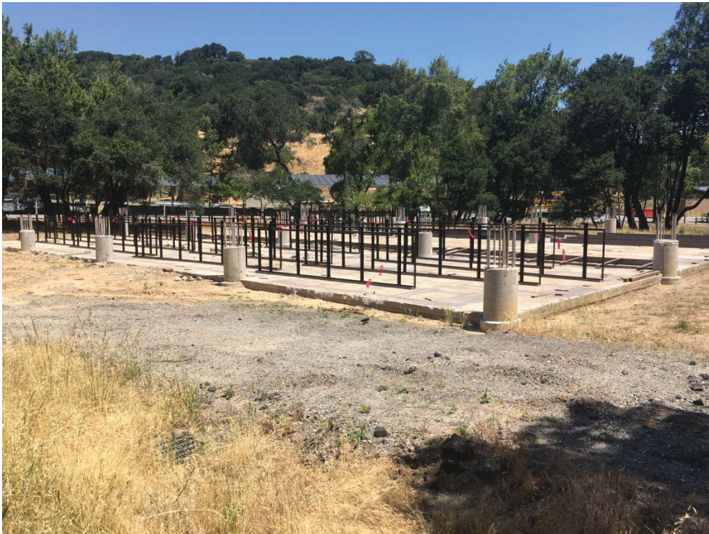
Photo 2. Jonas foundation with rebar (6/7/2018)
